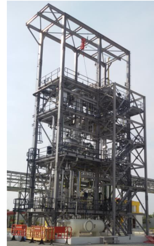
0.63 m diameter column at STCB (India)
